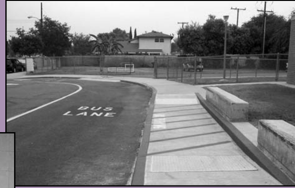
Parking Lot Improvements
