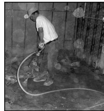
Construction work at Foothill High School
